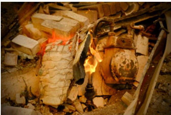
Gas Meter Rupture. Photo courtesy Don Silverek
